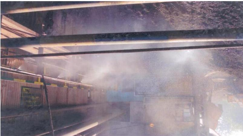
Water spray nozzles have been fitted at all transfer chutes and hopper to control dust pollution
